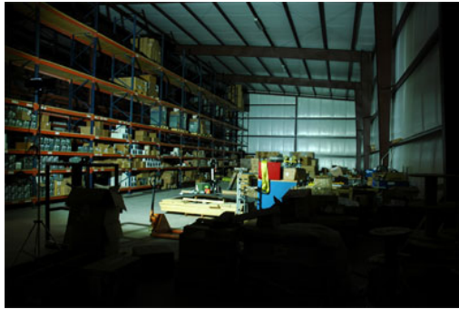
Same warehouse being illuminated by the LEDWP-400.
